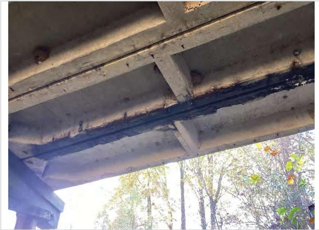
Span 1 PCCS 'H' spalling to steel with section loss
