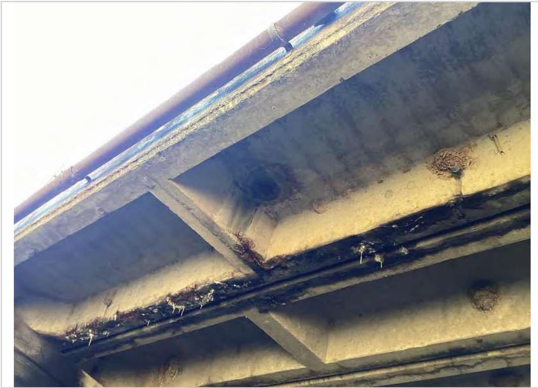
Span 2 PCCS 'A' spalling to steel with section loss
