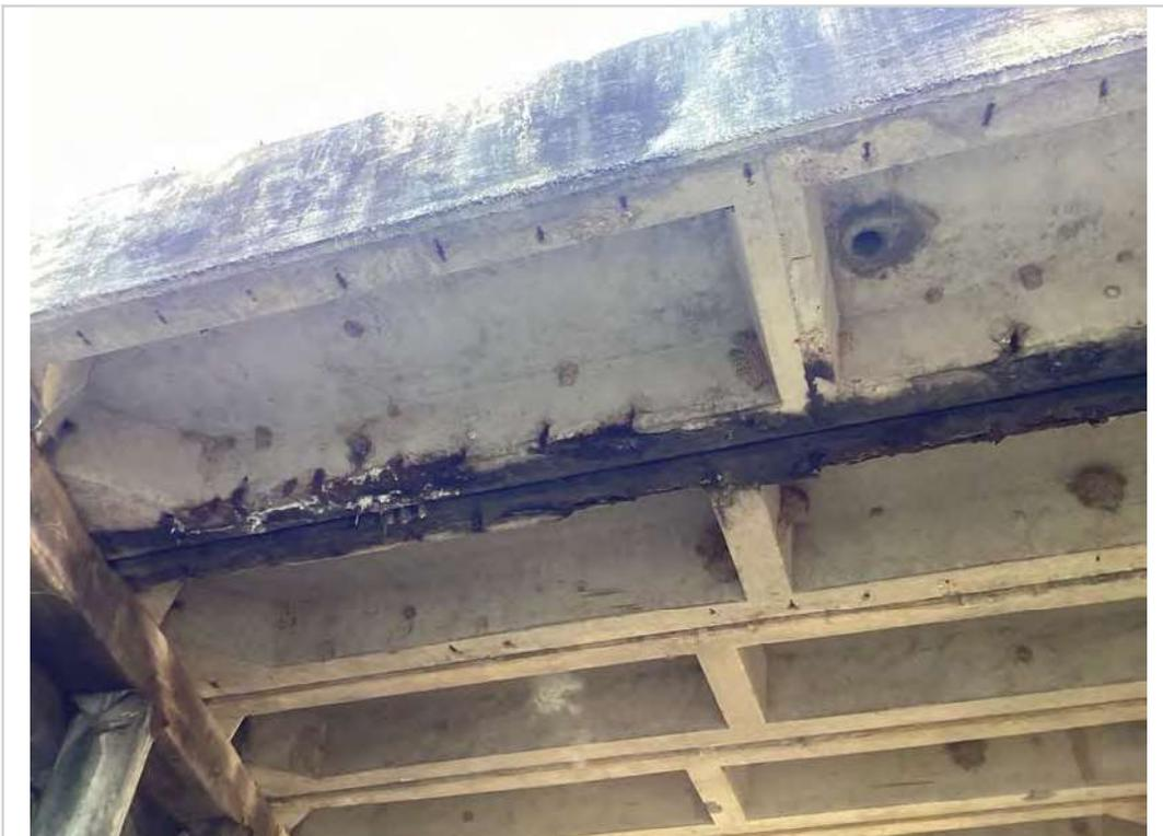
Span 1 PCCS 'I' spalling to steel with section loss
